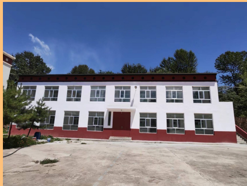
After the renovation
